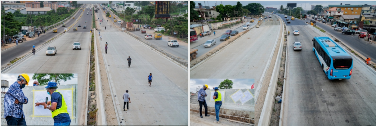
Ministry of works and housing, @tundefashola during the inspection of ongoing work on the reconstruction of Apapa-Oworoshoki-Ojota Expresswas in Lagos; Tue July 28, 2020. This is one of the Executive Order 7 roads. It is being rebuilt for the first time in 4 decades – as a concrete road.
