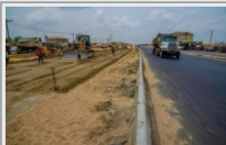
Reconstruction of Enugu-Port Harcourt Road (Section IV Aba-Portharcourt Expressway)
