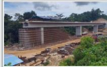
Construction of Ikom Bridge, Cross River state
